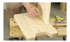
I used the front and back panels as gauges to locate the cleats that hold them to the ends. This avoids measuring errors.
